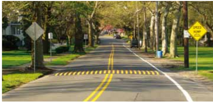
Traditional traffic calming device, parabolic in shape used to reduce speeds on residential roads.
