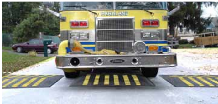
Series of small humps that slow cars while allowing emergency vehicles to pass.
