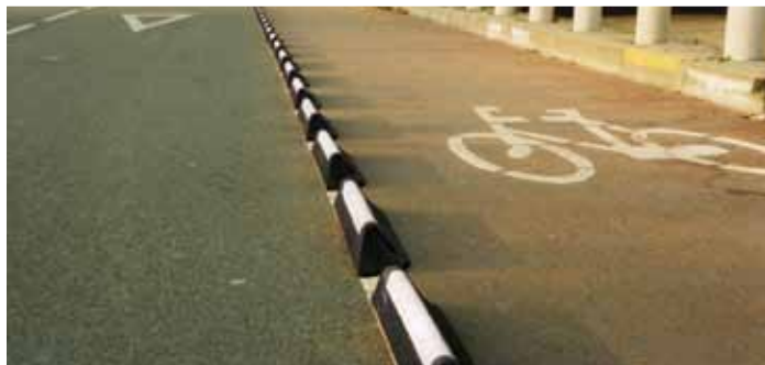
Bike lane curbing with a unique sloped profile to protect bicyclists.
