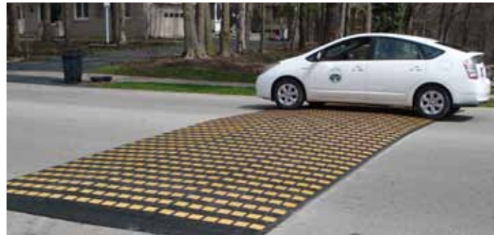
Flat topped traffic calming device used to slow cars more gradually than speed humps.
