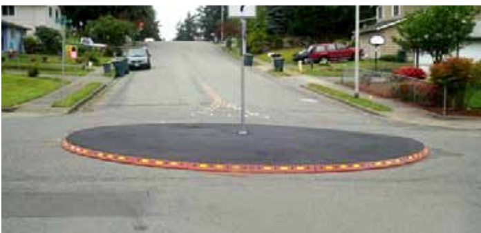
Flexible curbing units that can be used to create traffic circles and roundabouts.
